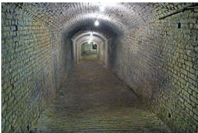
Gun ramp heading down to the right caponier.
